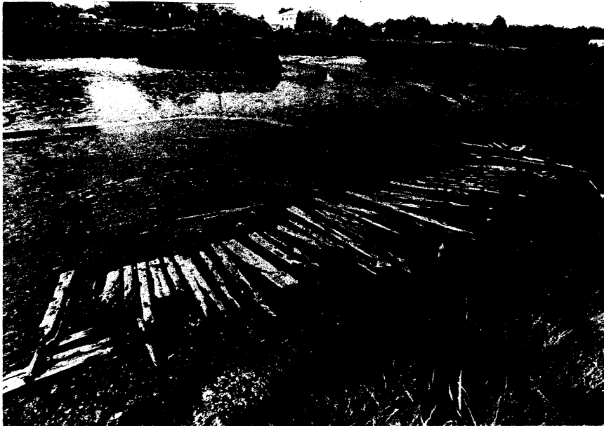
Figure 5. The derelict vessel prior to the excavation. To the right is the bow of the vessel. (Photograph by Patrick Grace)
