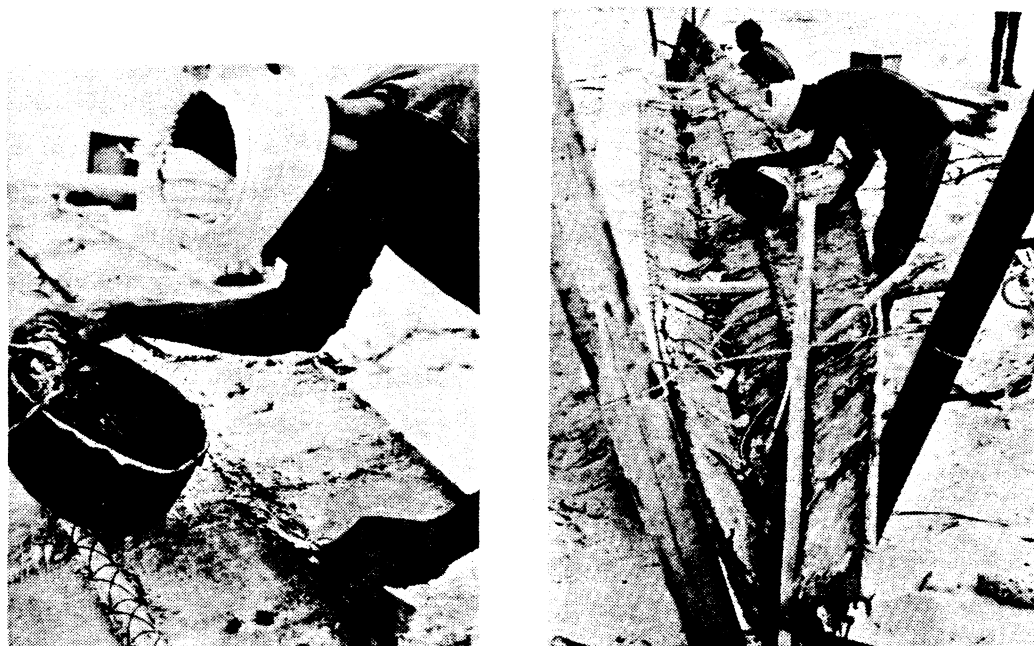
Figure 18. Pouring pitch into planking seam as part of caulking procedure.
