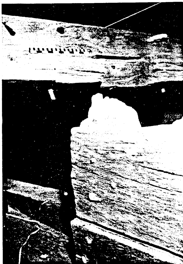
Figure 52. Mortices in the aft edge of the midship beam. Note forward end of centreboard trunk (below beam). (Photo by the author.)
