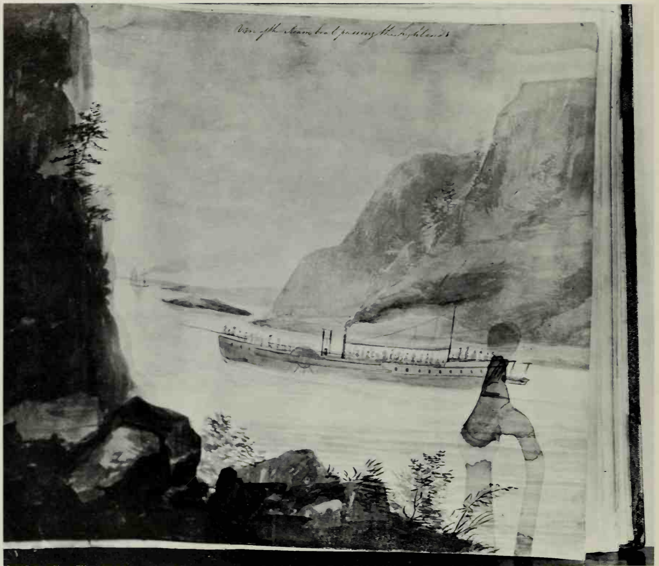
257. Fulton's first successful steamboat, popularly known as the Clermont , as sketched by the inventor himself. Her dimensions were: 140 feet long, fifteen feet wide, seven feet deep in the hold. The Survey of New York, accustomed to registering only sailboats, described her as "a square-sterned boat, has a square tuck:—no quarter galleries and no figure head." The engine, designed by James Watt, had one cylinder, two feet in diameter. The paddle wheels were four feet wide and fifteen feet in diameter.
