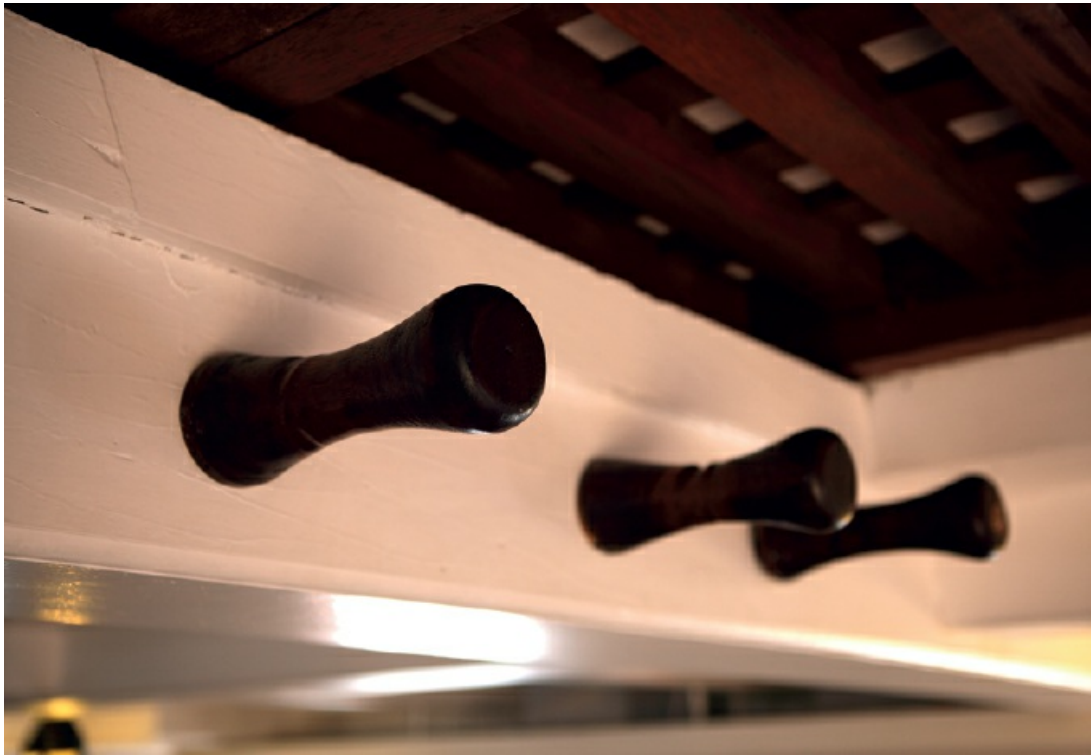
Belaying pins positioned in a deck beam adjacent to the grating over the waist which could be used to lash down spars or any other gear stored in the waist.
