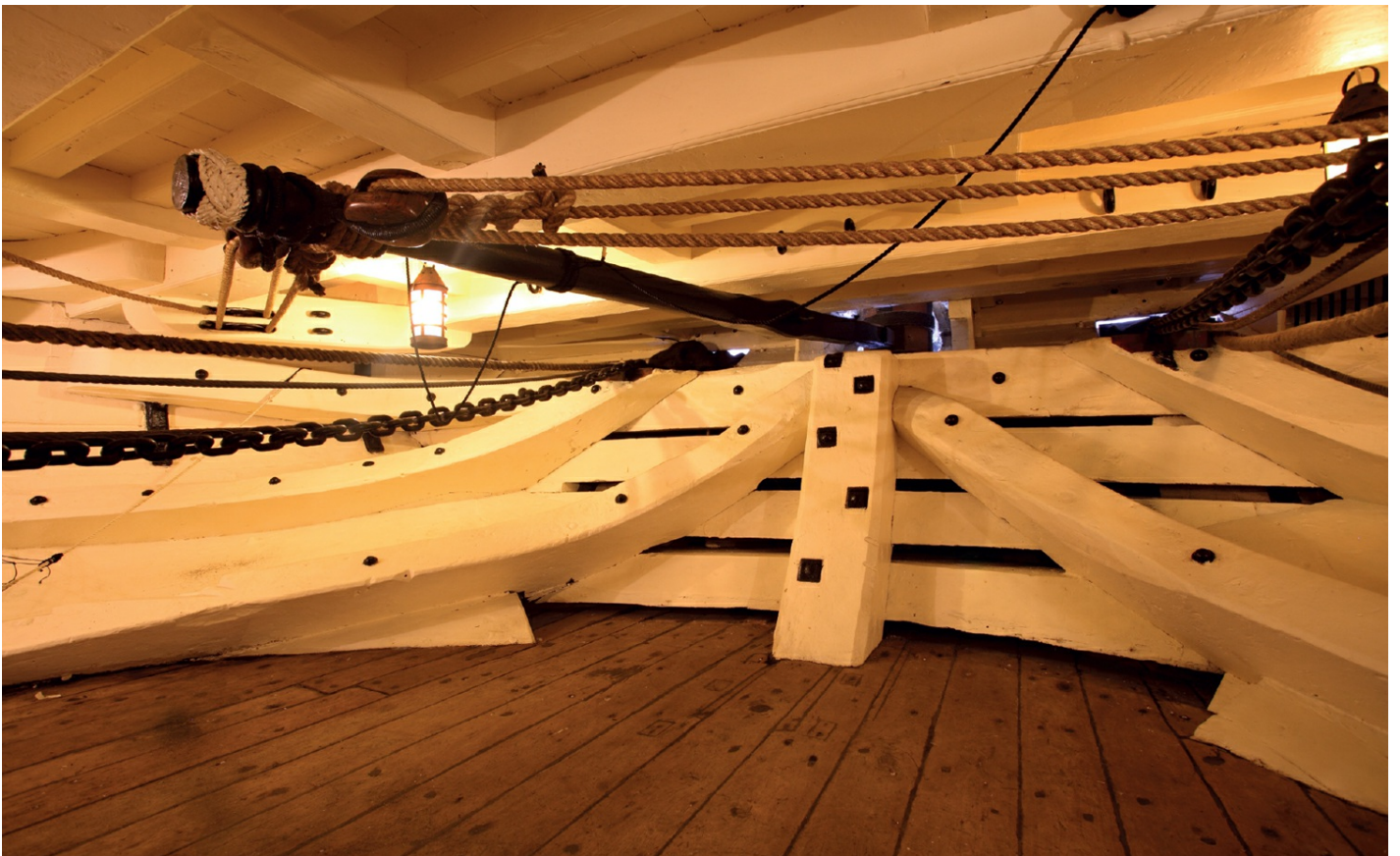
The Seppings iron tiller located above the bread room aft of the wardroom. The chains visible passing under the deckhead are the modern mooring chains, but otherwise this compartment is much as it would have been in 1817. The large curved timbers sweeping up to the transom timbers are the transom knees, or sleepers. The upright timber is the stemson knee attached to the stempost on which the rudder is hung. The lines controlling the tiller lead to double sheaves (left of photo, under the tiller) greatly increasing the purchase.
