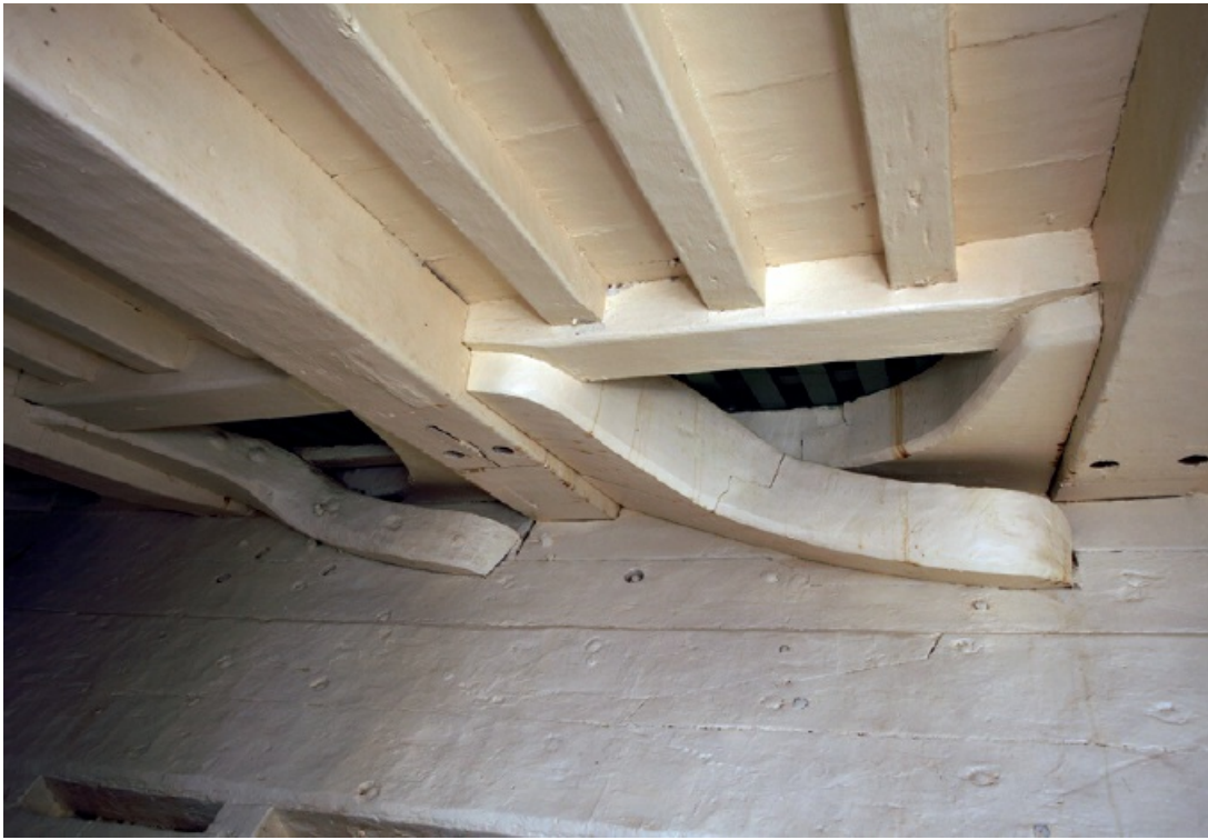
The port side of the hold showing the lodging knees and beams of the orlop deck. The lodging knees are ingeniously fashioned, straight and curved, to fit in the narrow space between the beams. The carlings, running fore and aft, are neatly fitted between the beams and the knees.
