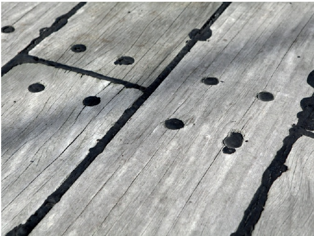
A close up of the deck planking and the caulking between the planks. Caulking made the seams watertight and consisted of unravelled rope called oakum hammered into the seam followed by hot pitch poured in to complete the joint. Picking oakum, as the process of unravelling was called, and then selling it, is the origin of the saying 'money for old rope', although it was by no means as easy as the modern usage implies.
