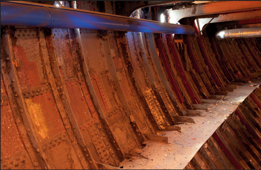
Detail of the remains of one of the original decks left in as a stiffener along the ship's side after conversion to a pure cargo-carrying sailing ship.
