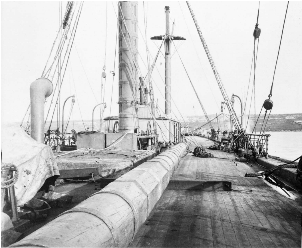
This shot could be earlier than the one above as work is clearly in progress, but the main yard seen rigged above is here lying on deck. There remains some running rigging still to be seen and the canvas covers would not have survived long after being hulked. (The SS Great Britain Trust)
