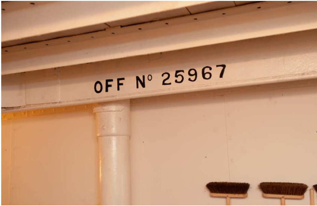
The ship's official registered number 'carved' on one of the iron main deck beams. This particular beam was once part of the frame of the central cargo hatch but has been repositioned during restoration, and is now at the after end of the steerage pantry.
