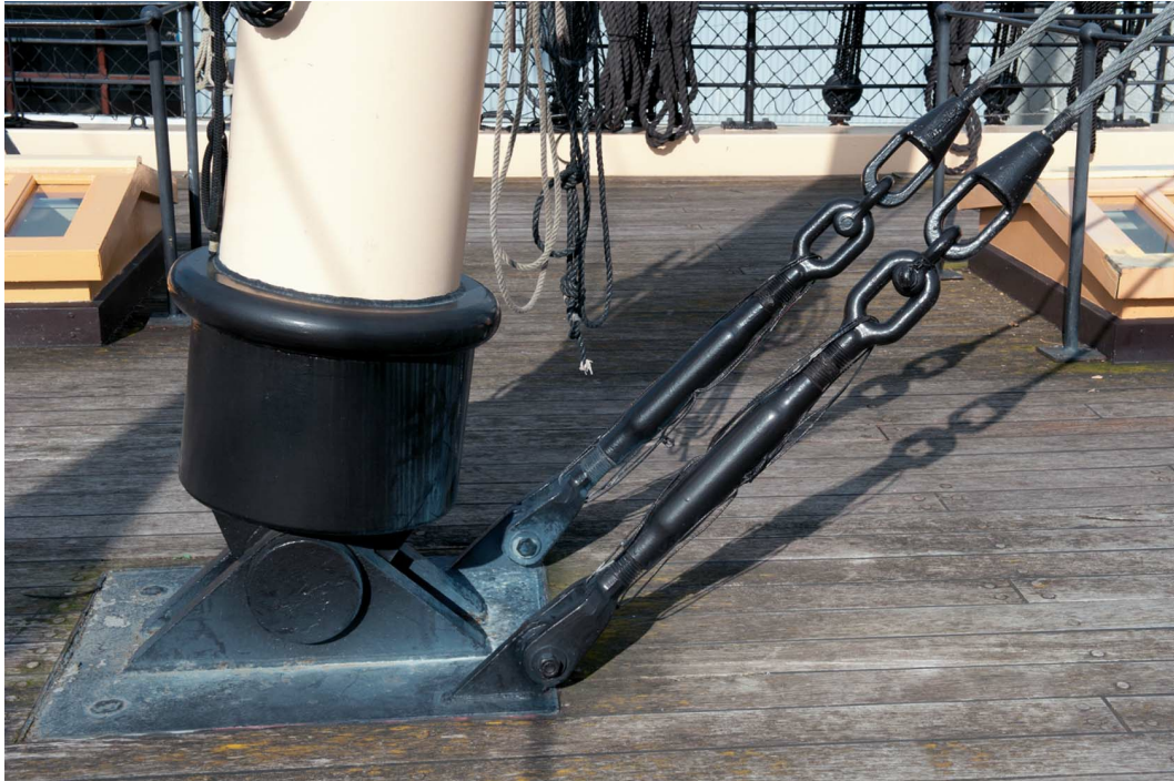
The hinge at the foot of No 5 mast. The two forestays visible here are those from mast No 6. In another engineering solution unique to the ship, the upward force of the stays counteracts the downward load of the mast to minimise the strain on the deck structure.
