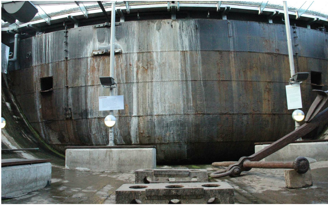
The 1928 caisson in place. To ensure the dock is as watertight as possible another gate has been built outboard of this, rather than try and repair the caisson which would have meant taking it away just when it was most needed! Note the modern additions of supports for the glass roof. ( The SS Great Britain Trust )
