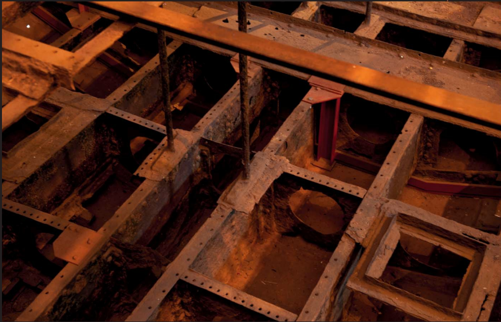
A closer look at the enormously strong 'egg-box' structure worked into the bottom of the ship. This would have been mainly plated over at the start of her career to form the double bottom.
