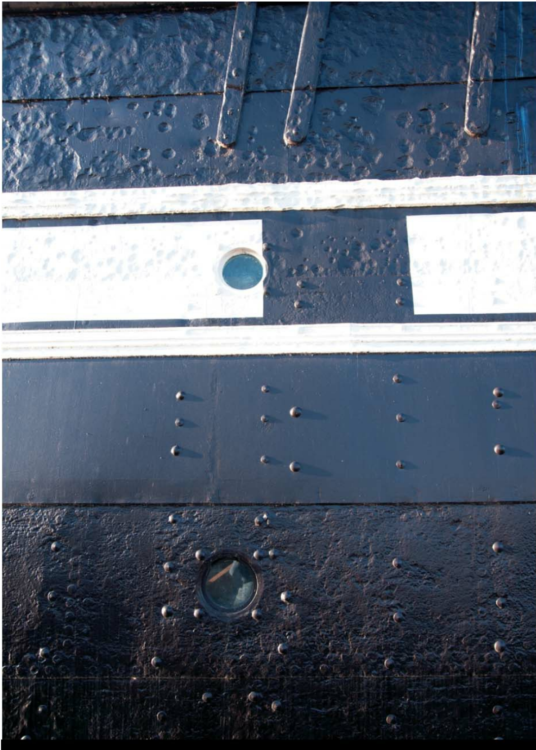
The second row of portholes lit the saloon deck below.
