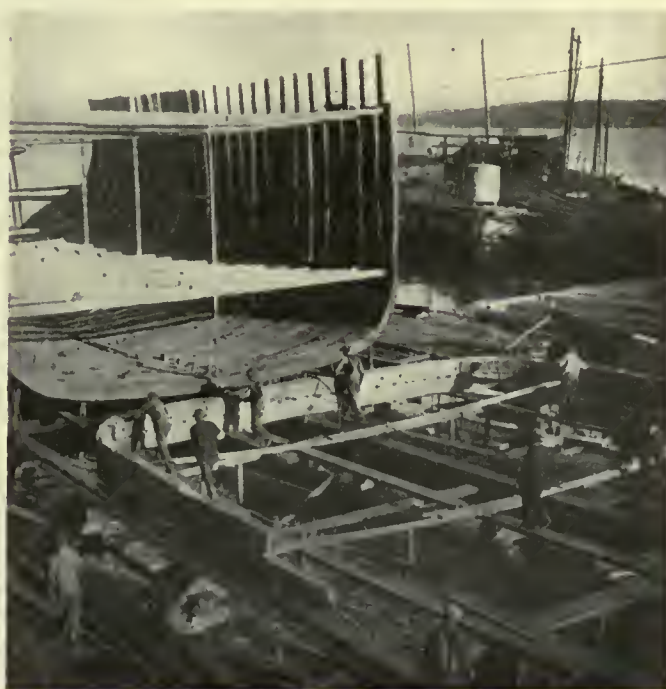
Fig. 76a. Erecting a Midship Frame
