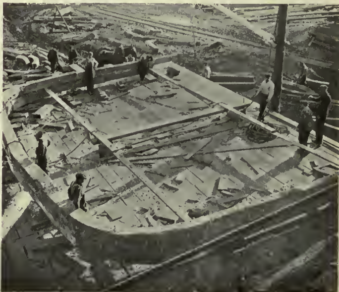
Fig. 75. Assembling a Midship Frame
