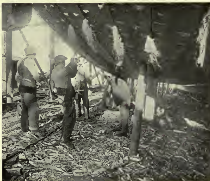
Fig. 93. Caulking Bottom Planking
