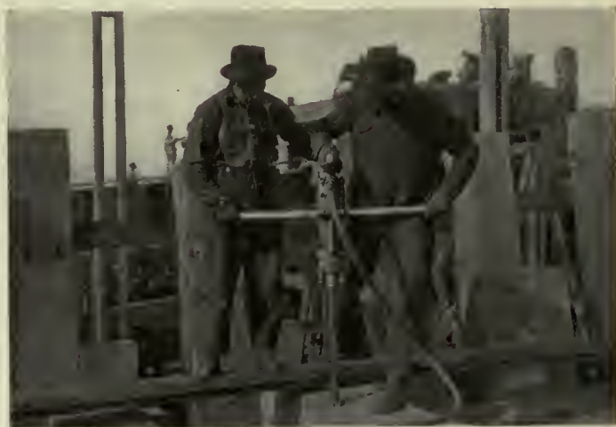
Fig. 81a. The Pneumatic Drift Bolt Driver Hammering Home a Long 1 1/4-In. Bolt Through a Deck Beam and Its Supporting Sturdy Sill. The Bolt Disappears Into Its Hole With Astonishing Rapidity
