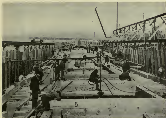
Fig. 53. Deck Framing and Waterways
