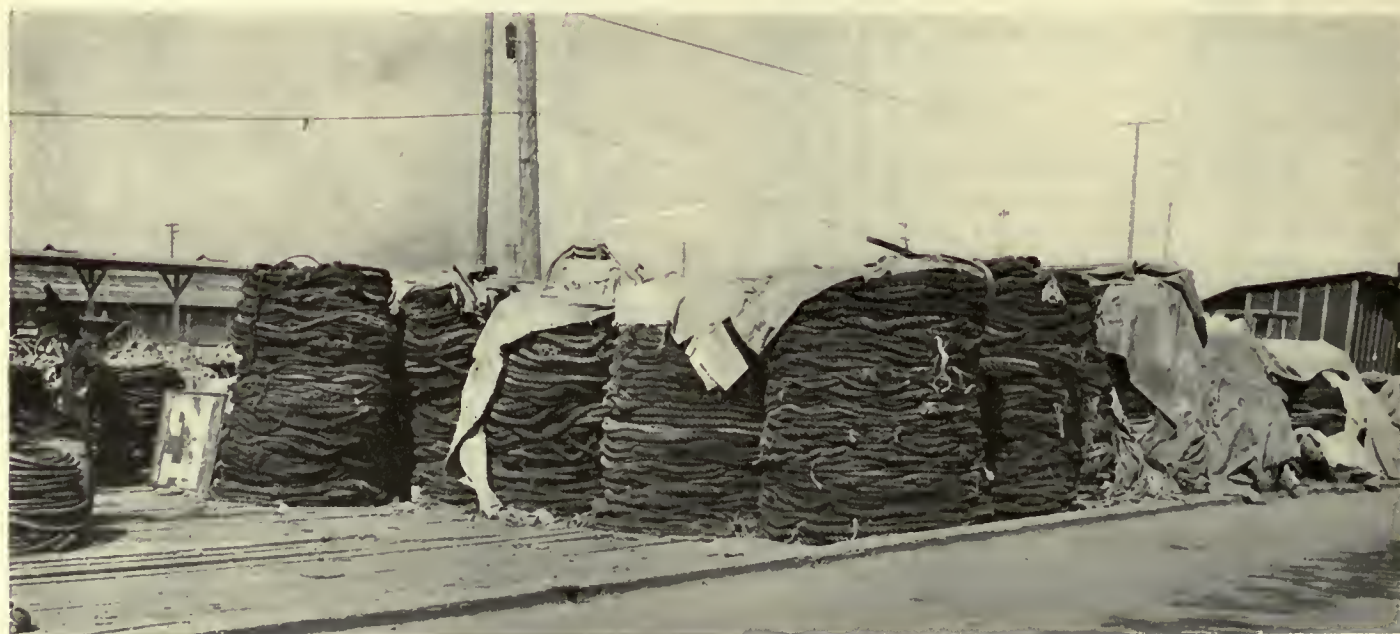
Running Rigging Ready to Reeve Off
