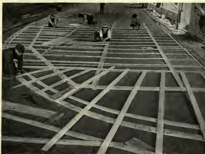
Fig. 73. Mould Loft Work
