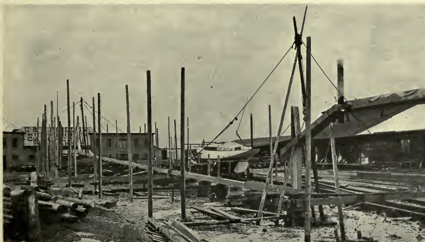
Fig. 82. Setting Up the Stern
