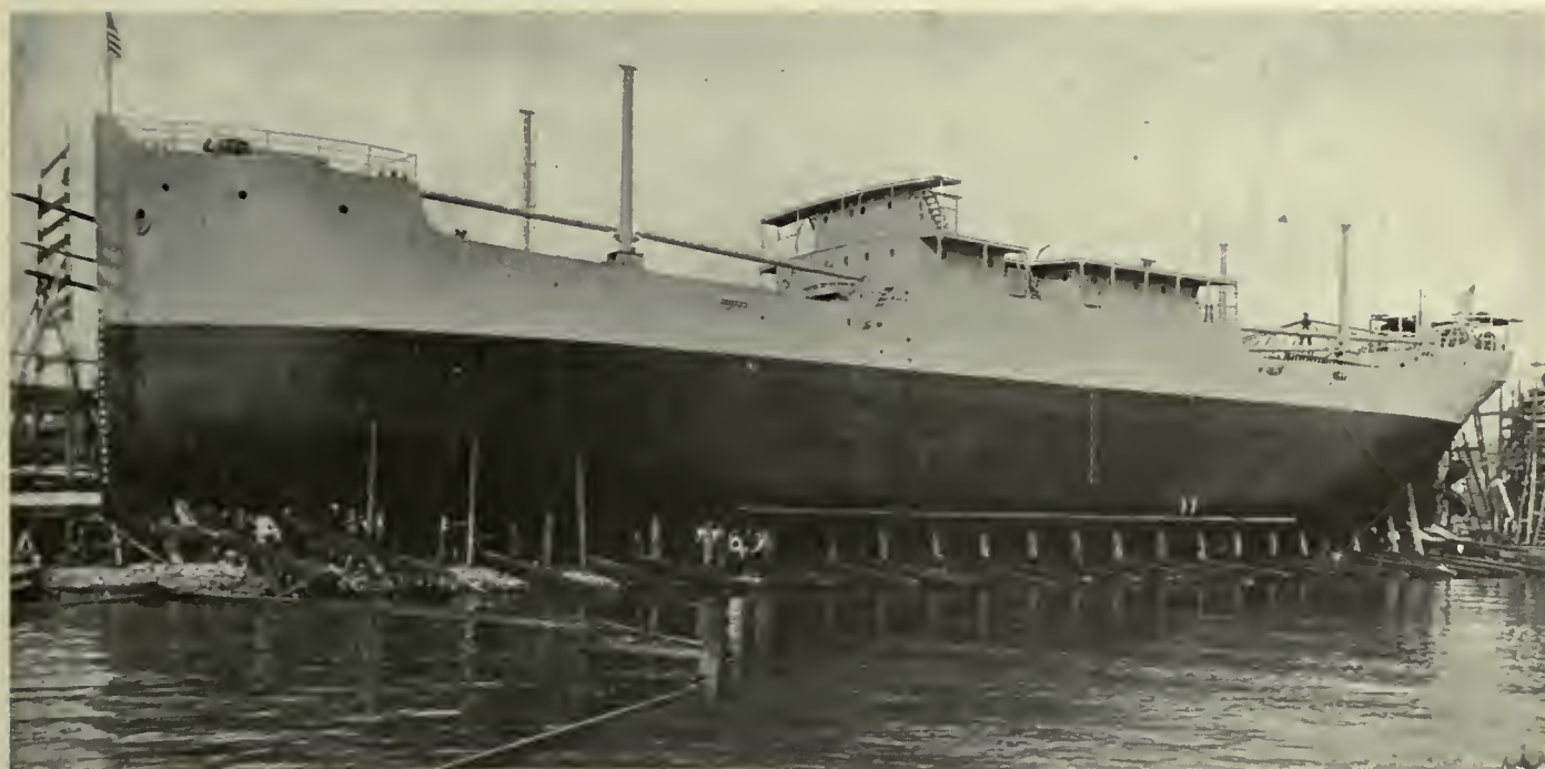
Fig. 68. Lake Silver. at the Great Lakes Engineering Works at Ecorse, on the Ways Ready For Her Sideways Plunge
