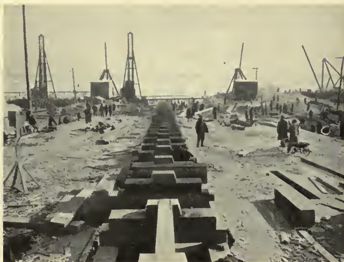
Keel Blocks Being Laid
