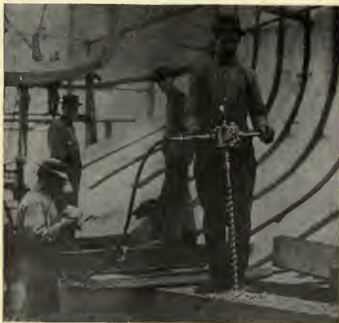
Fig. 81. The Little David Pneumatic Boring Machine Makes Light Work of the Deep Holes Required in the Giant Keelsons. The Operator Has to Have Only a Straight Eye and a Steady Hand, For His Task Is But to Guide the Tool
