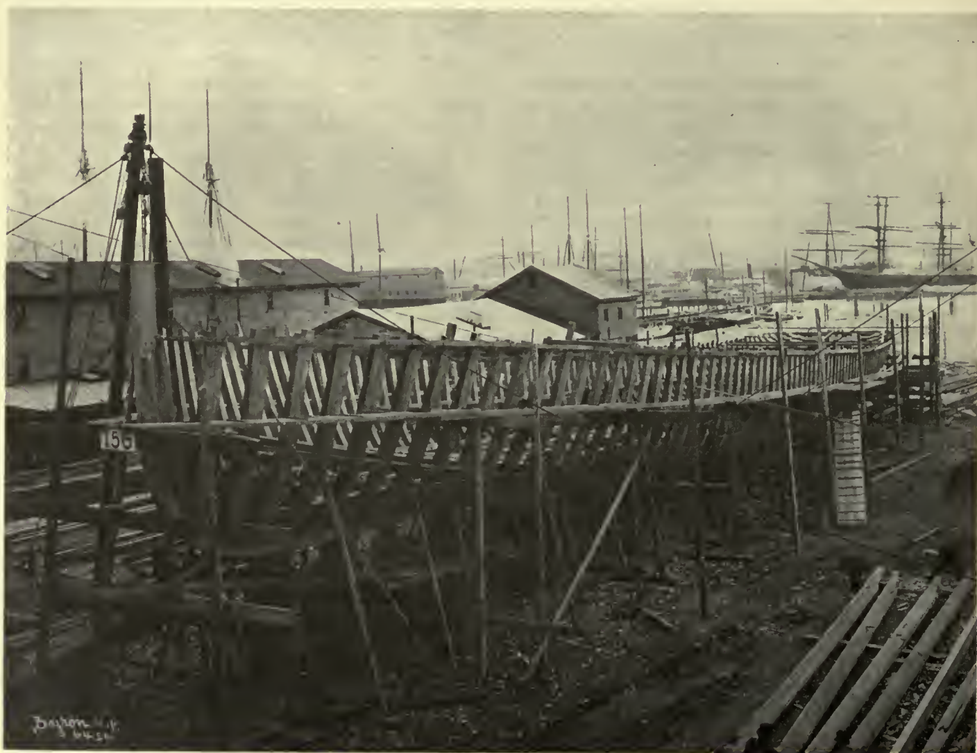
Fig. 90. Framed Ready For Sheer
