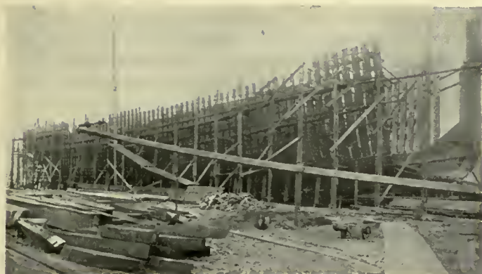
Fig. 79. Stem, Deadwood and Frame Set Up
