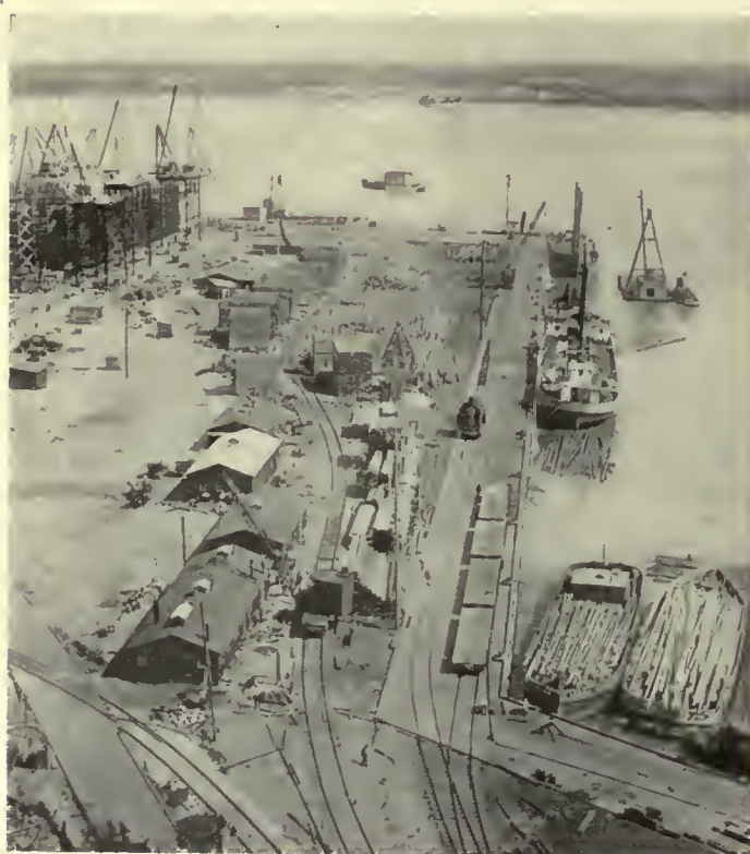
Fig. 72. Traveling Hoists and Tracks in Shipyard
