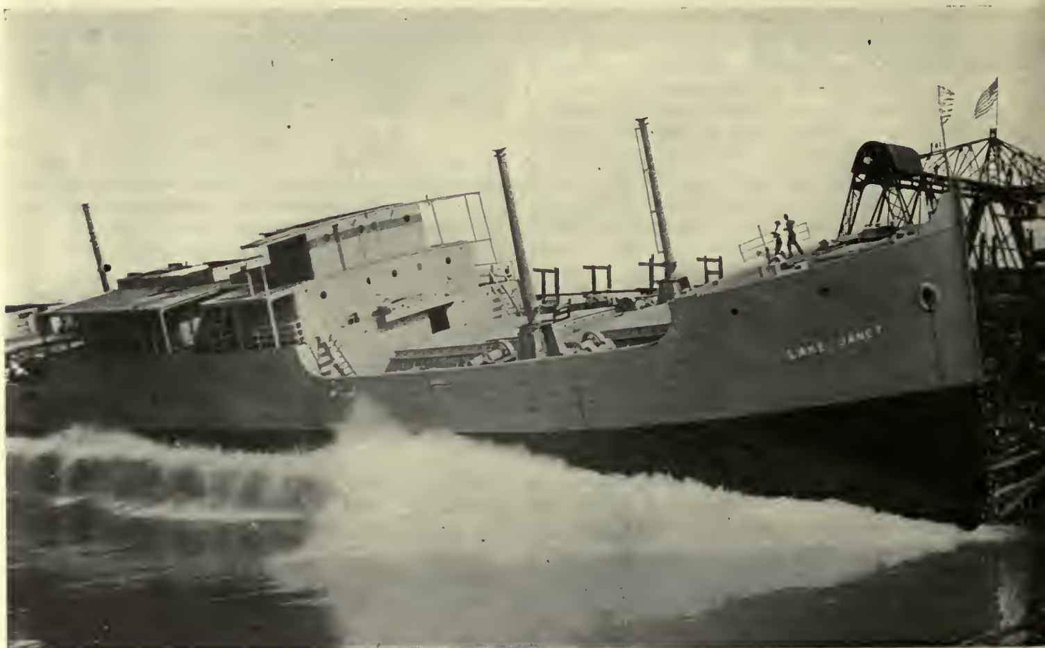
Univ Calif - Digitized by Microsoft® Fig. 70. A Broadside Launching at the Ecorse Yard, Great Lakes
