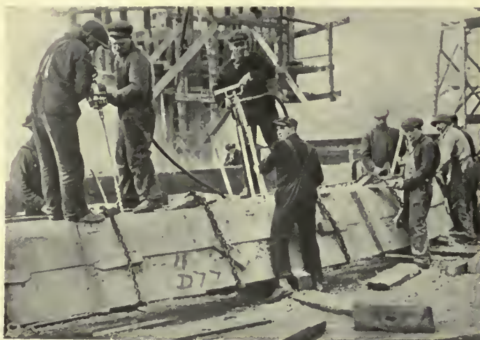
Fig. 74. Assembling a Frame
