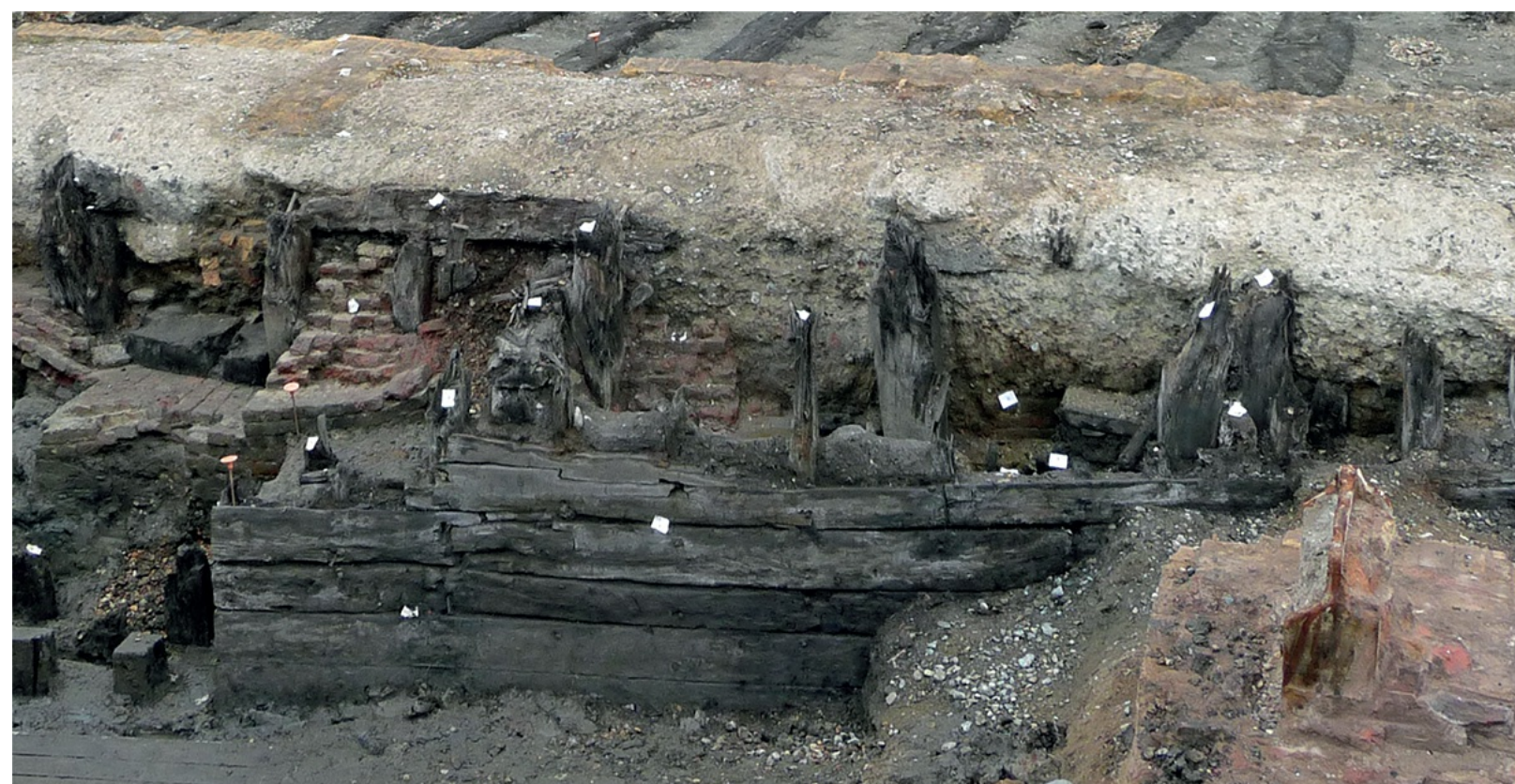
Part of the side of a broken-up ship at Deptford dockyard as revealed by recent excavations. Parts of ships were often used in dockyard buildings and docks Author.
