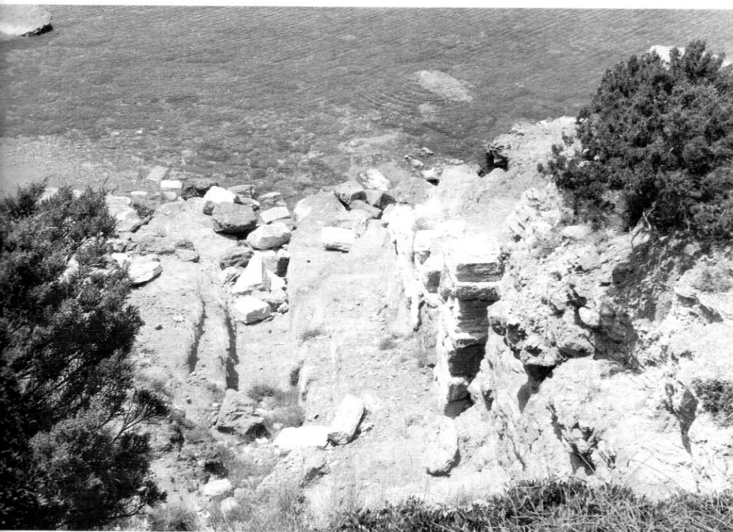
The remains of two small rock-cut slips at Sunium. The angle of the ways is very steep at about 1 in 3.5. (David Blackman)
