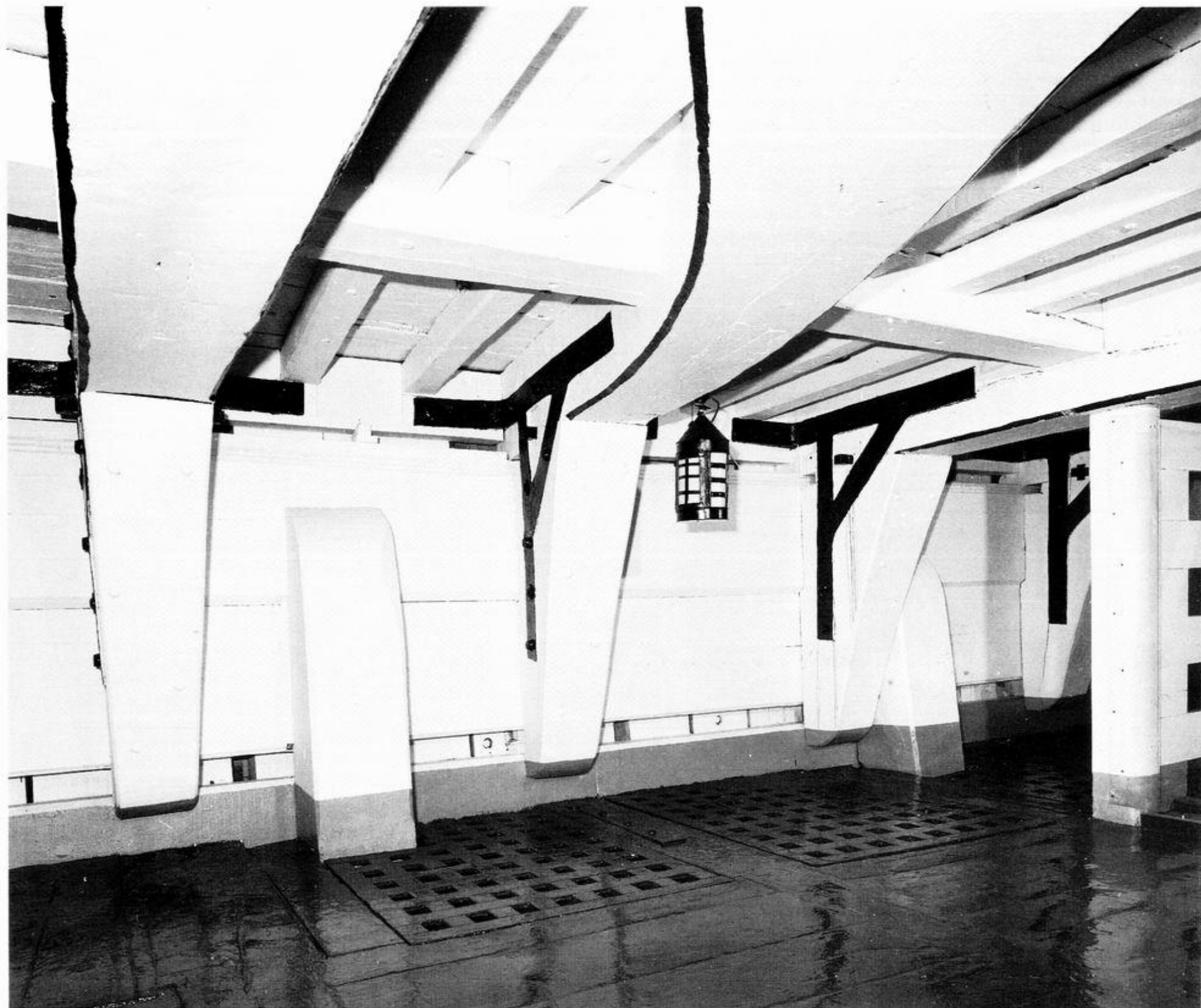
Victory. The orlop deck with its gundeck beams, beam arm and associated carlings and ledges, and chock knees braced with Roberts iron plate knees. The deck clamp at this point is exceptionally deep in order to support the weight of the gundeck. The spaces between the strakes of planking are to give ventilation to the timbers (or frames) visible in places. The two vertical timbers are the heads of the riders. Note that the orlop planking is made in short lengths set between and level with the upper edges of the orlop deck beams.
