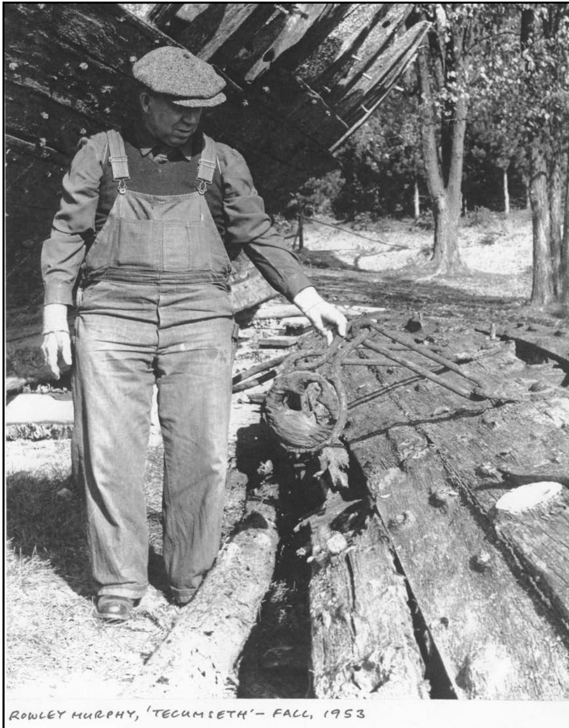
Figure 31. Historian Rowley Murphy holding chainplate on Tecumseth in 1953. (Photograph: John R. Stevens.)
