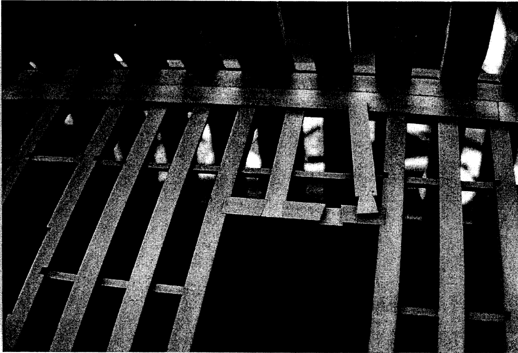
Figure 57. Deck framing installed. Note the method of dovetailing the ledges into the hatch carling. Photo by G. Grieco.
