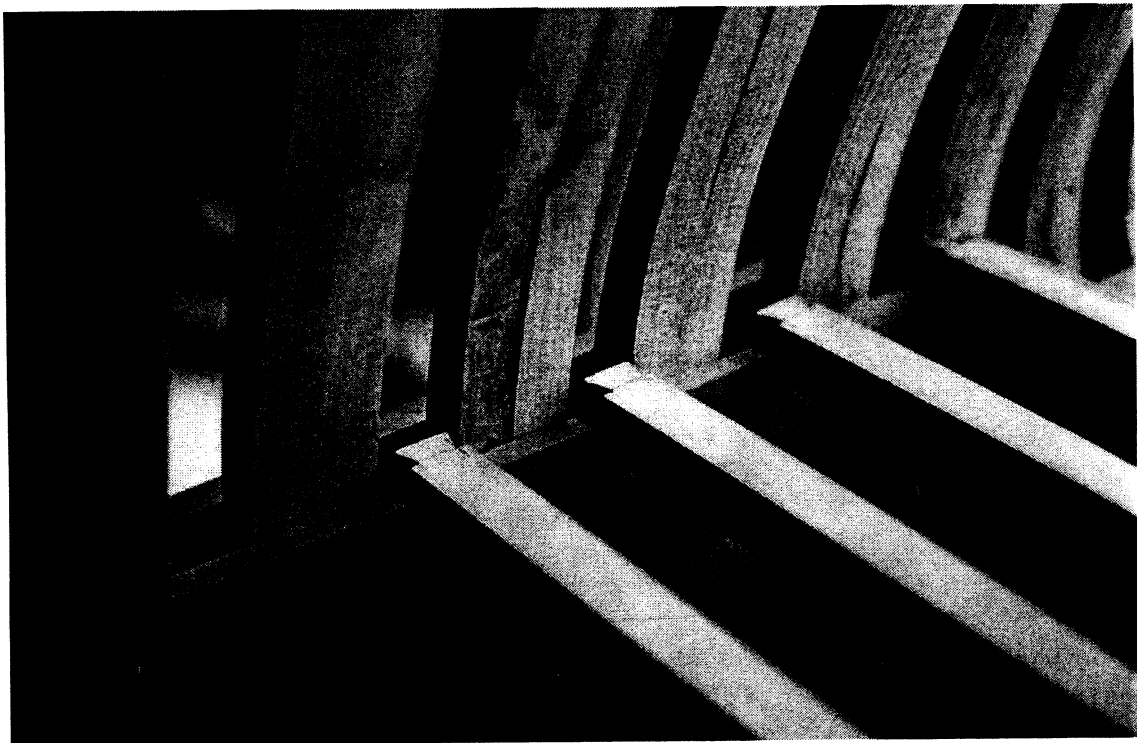
Figure 54. Dovetailing of beams into the beam clamps. Photo by G. Grieco.
