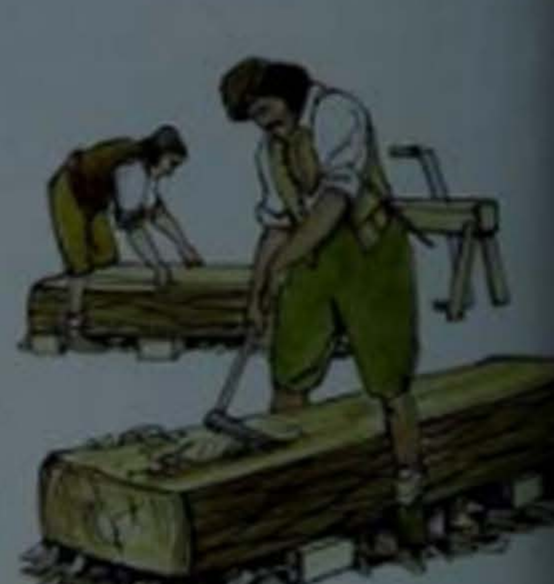
Back to work. The new timber is shaping up nicely, its surface smoothed by strokes of the razor-sharp adze.
