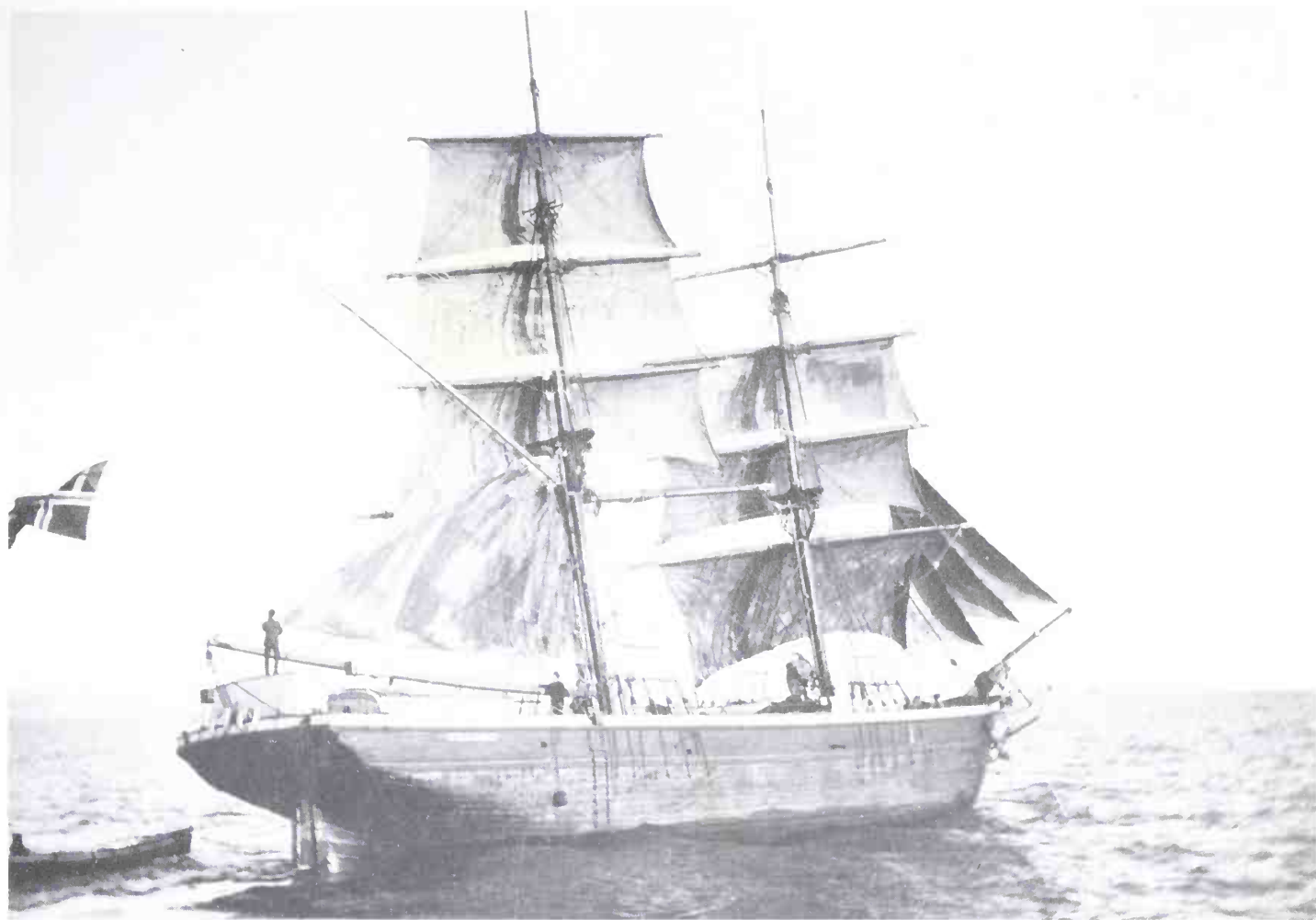
Fig 83. The Tromsø built in 1862 under easy sail in ballast. When photographed late in their life, many brigs no longer set royals. (Nautical Photo Agency)
