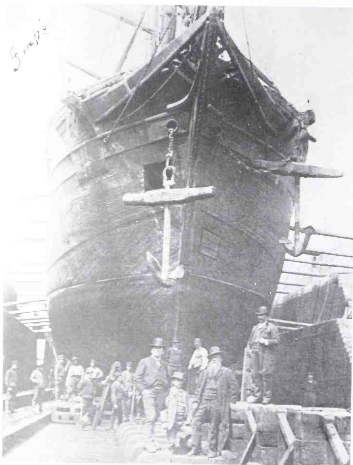
Fig 147. The bow view of the Impi illustrates a wooden hull with doubling, and upper and lower timber ports; also the trail boards and brackets. This barque was built at Brahestad, Gulf of Bothnia, Finland, by E Klubb in 1868; Bureau Veritas (1884) gives her measurements as 43.6m × 10.4m × 6.24m and 637 tons. Photograph by George Gjersoe. (David Clement Collection)
