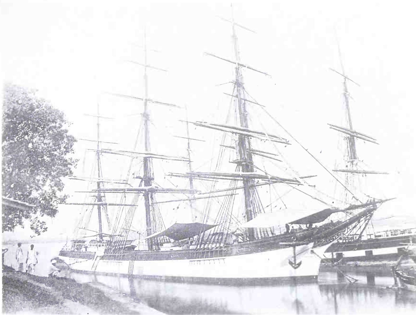
Fig 228. Photographed at her moorings in Calcutta in 1870 when only two years old, the Augusta still has the trappings of a new ship of the sixties with all her stunsail booms aloft, with the exception of the fore topgallant yard, although the boom irons are fitted. Beyond is one of Donald Currie's ships, identifiable by having the black ports 'upside down'. I am grateful to Andrew Nesdall for this photograph and for data on Currie's ship. (Andrew Nesdall)
