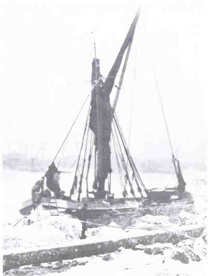
Fig 135. In this severe frost in January 1881 when blocks of ice were piled high on the banks of the Thames, the spritsail barge Collingwood was photographed on the western side of the Isle of Dogs. There were two barges of this name and the likeliest was the one built at Grays in 1863 of 38 tons and owned there. The photograph shows tiller steering, a round stern, wooden stay fall blocks, a short mizzen and the topmast housed. I am grateful to Jocelyn Lukins for giving me this picture.
