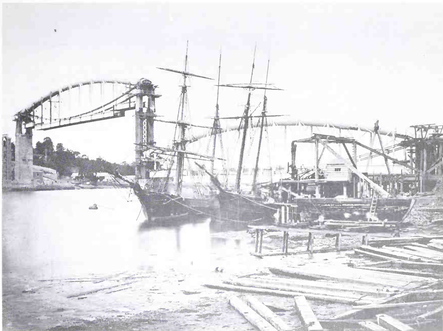
Fig 105. Brigantine and schooner lying at Saltash in 1858 while behind them Brunel's tubular suspension bridge has had one of the spans erected. (Museum of British Transport)
