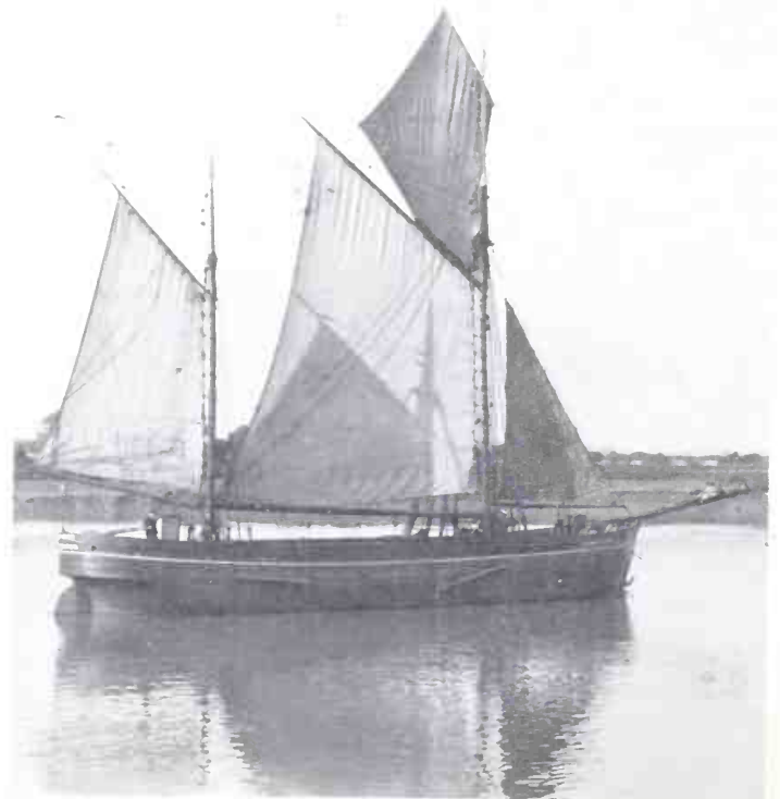
Fig 133. Here is the ketch-rigged Fanny Jane in the River Parrett near Dunball below Bridgewater . She had been built there in 1858 and had a tonnage of 65 and was still steered with a tiller when W A Sharman took this photograph. The foresail set on a boom. (MacGregor Collection)
