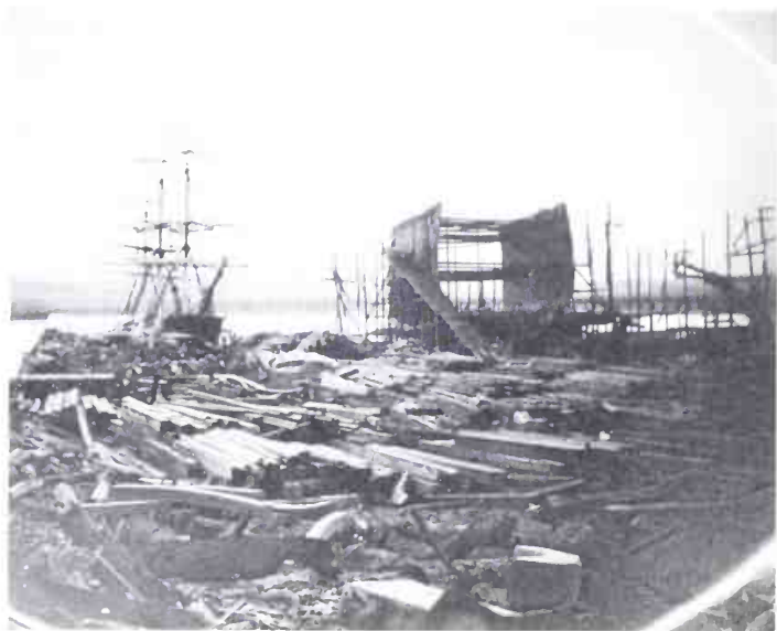
Fig 44. Donald McKay's shipyard at East Boston, probably taken in the 1850s. All the midship frames have been erected for some vessel but the stem and sternpost have not yet been set up. In the foreground are stacks of timber some of which is 'grown'. (Peabody Museum, Salem)
