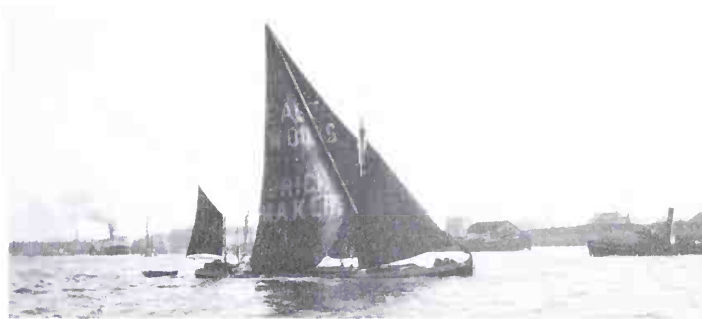
Fig 304. An unidentified stumpy barge bearing the words 'EAST-WOODS BRICKMAKERS' on the spritsail. She is deeply laden with the bulwarks still above water amidships, which was a common sight. This one has a steering wheel. Photograph by Basil Lavis or a copy negative by him. (MacGregor Collection)
