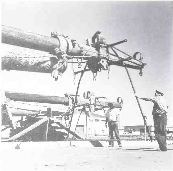
Fig 215. The Star of India, built at Ramsey, Isle of Man, in 1863 as the ship Euterpe is now preserved at San Diego, California. This photograph shows the restoration of her masts in the early 1960s, with the fore- and mainmasts propped up on the quayside. The wooden topmasts have been sent down: the topmast cap is on the right; next come the iron spreaders and crosstrees, and then the wooden trestletrees; the parral for hoisting the upper topsail yard is close against the iron lower mast cap; the paint is peeling from the iron lower mast. The scale is provided by the men. (Photograph by Karl Kortum)
