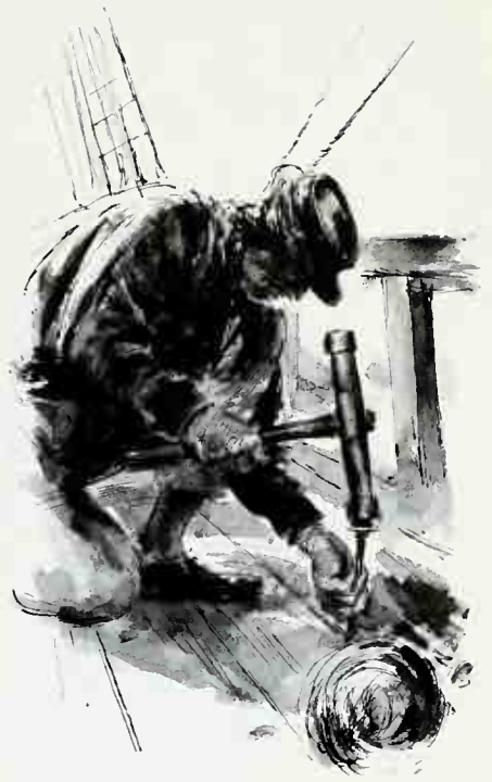
The carpenter caulking deck seams.
