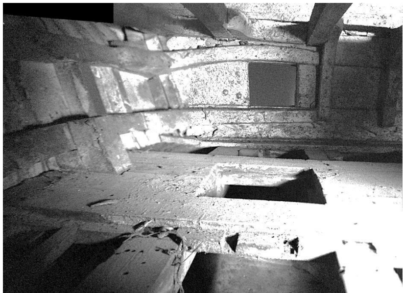
Fig. 19: View of the lower-deck structures at the stern, as seen from the last starboard-side gun-port. Ditta 2014.
