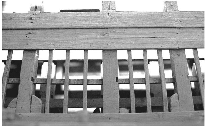
Fig. 25: Detail of the carlings/ledges system on the upper-deck. Ditta 2014.
