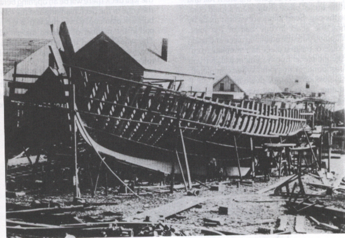
Schooner in frame in the last century at Gloucester, Mass. Ribbands are keeping the frames aligned as planking begins—the garboard and next two planks are already in place. This scene is so typical of ship construction, that it could have been at any of the countless yards along the coast.
