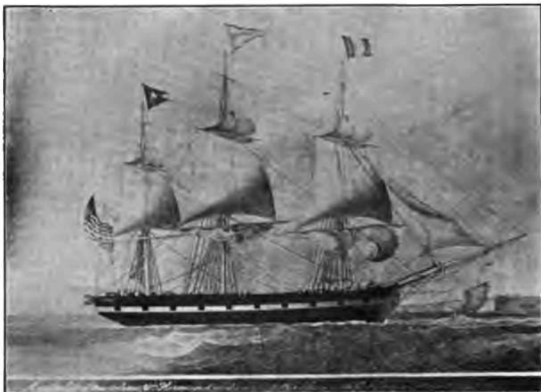
[17] "AUSTERLITZ," CAPT. WILLIAM HAMMOND OF MARBLE- HEAD, MASTER, ENTERING THE PORT OF HAVRE, JANUARY 9, 1834.
