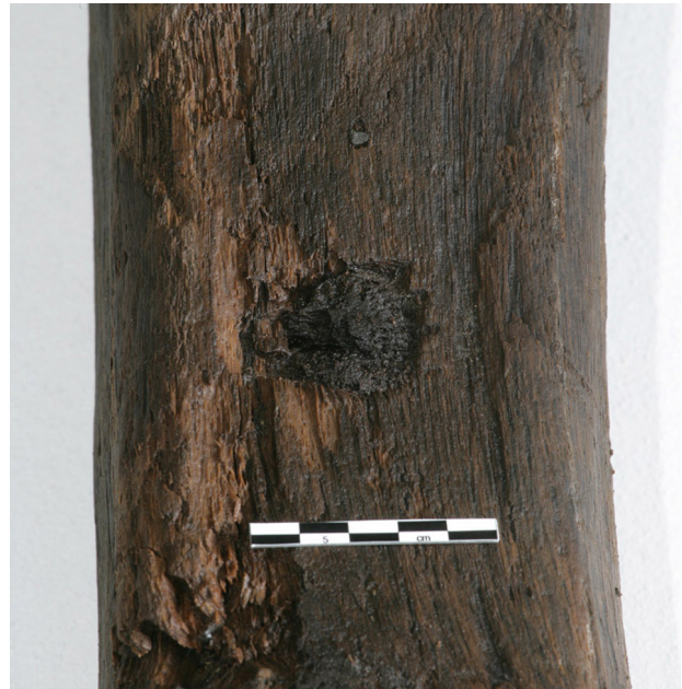
Figure 3-31: Detail of roughly cut treenail rebate (Brogan 2009)
